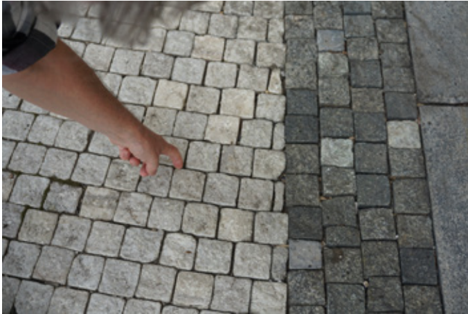
Figure 10. Kovanda points at a spot where the installation happened. Photograph by Maruška Svašek, 2017.
